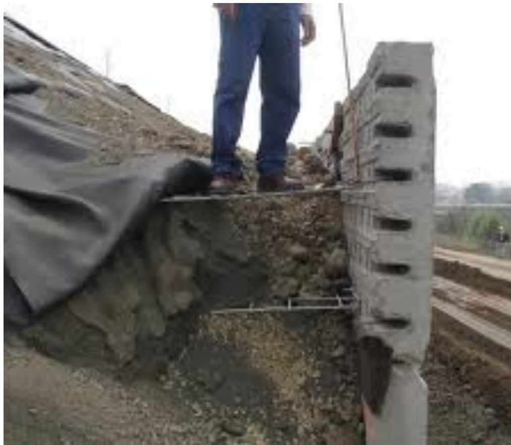
Galvanised steel geogrid (mesh) or strips
